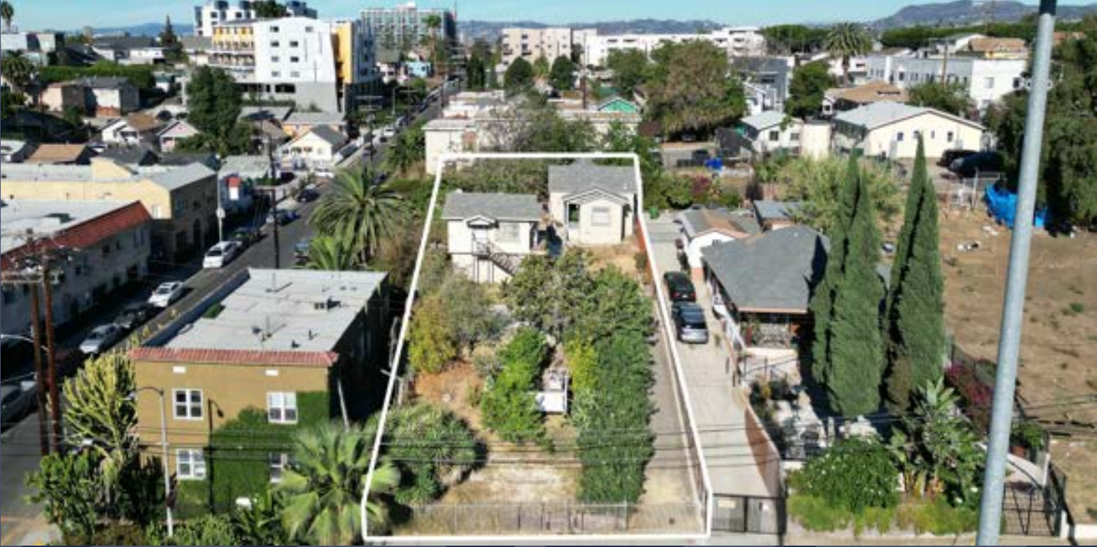
DRONE SHOT OF FRONT
